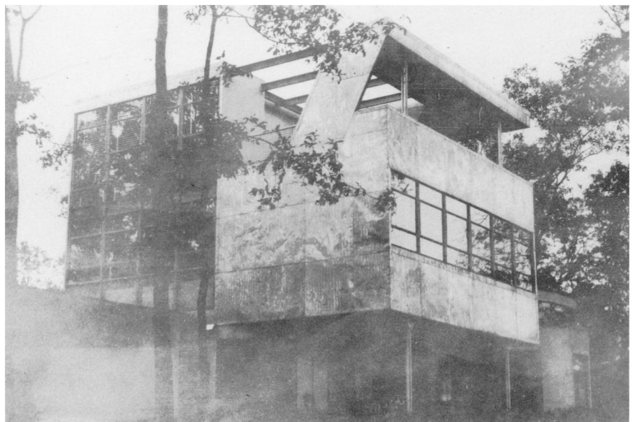
5. View of southwest corner with Harrison's additions on either side of garage, ca. summer 1931
