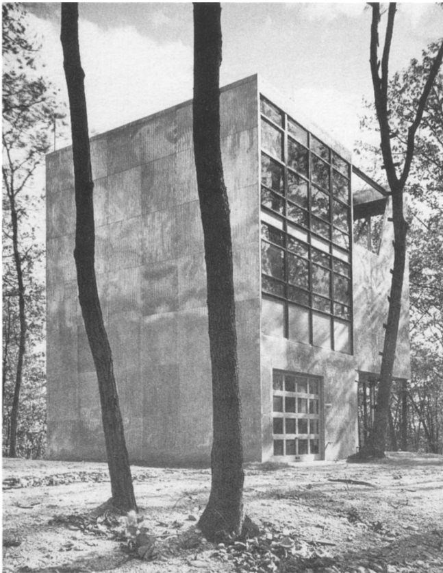
24. View of northwest corner
